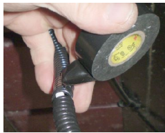
TAPE THE SPLIT LOOM (NOT SUPPLIED)
